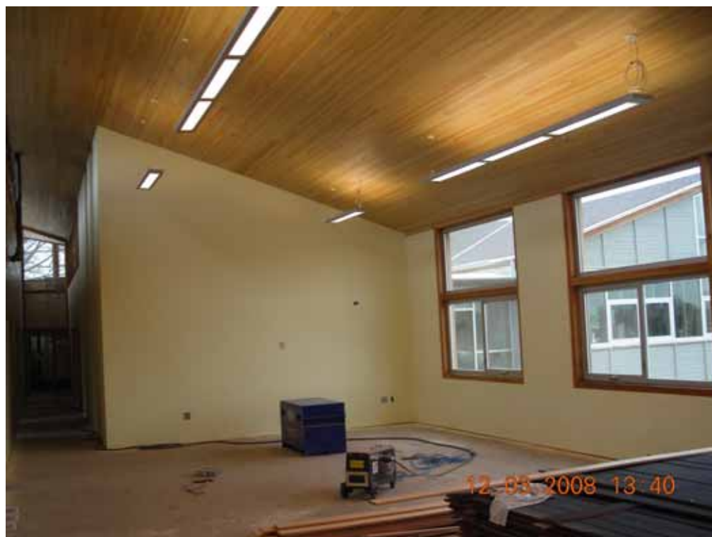
Main open office area looking southeast.
