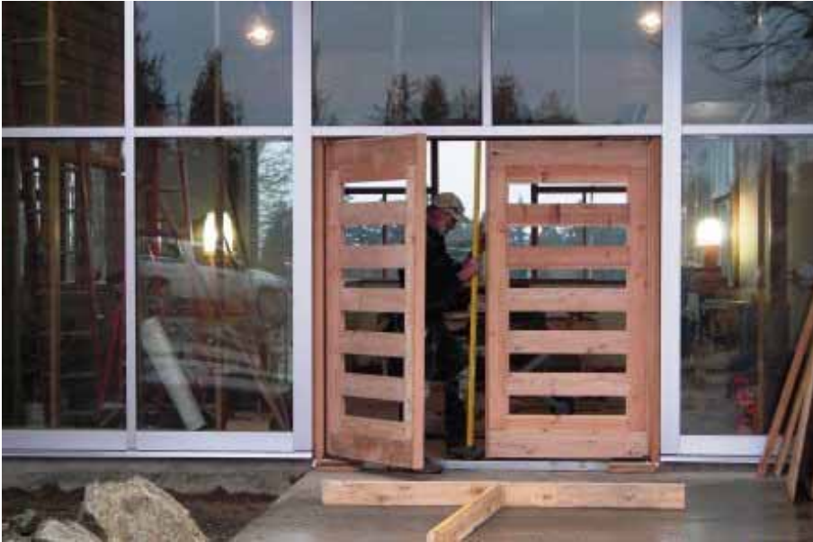
Front door assemblies being hung for fitment measurements, prior to glazing and applied finishes.
