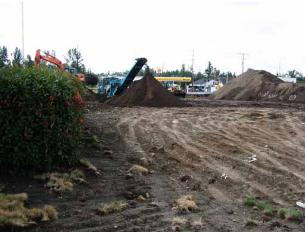
Separating Top Soil on front portion of the property near Meridian
