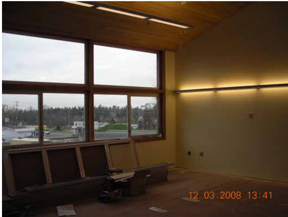
Main open office area looking southwest.
