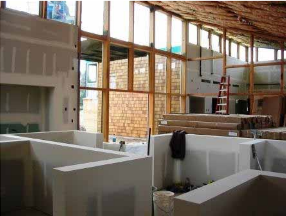
Front Desk/Counter Facing the Front Door
