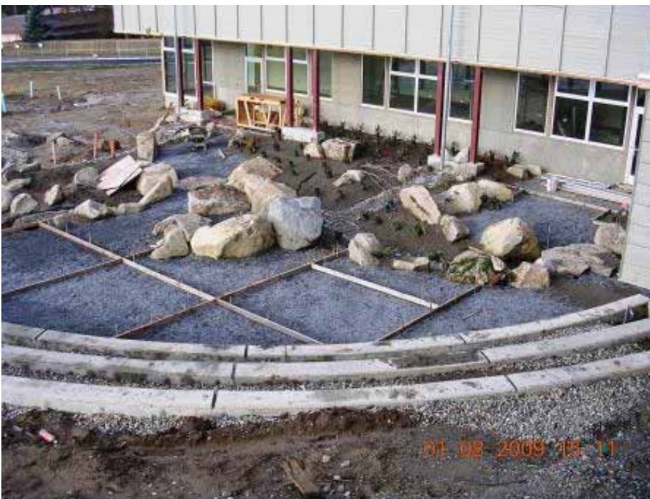
Lower courtyard formed for final paving and landscape materials being located in planting beds.
