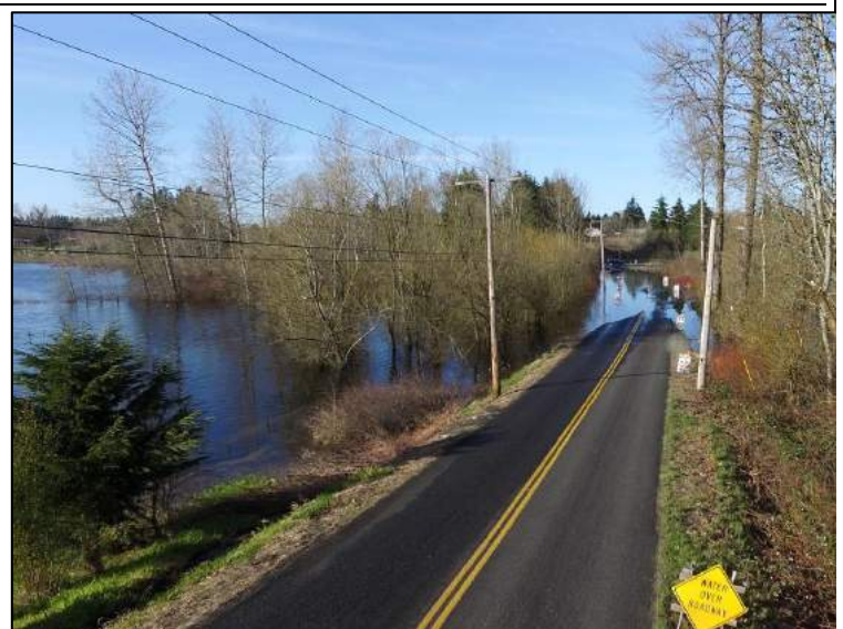
Edgewood Bowl pothole flooding
