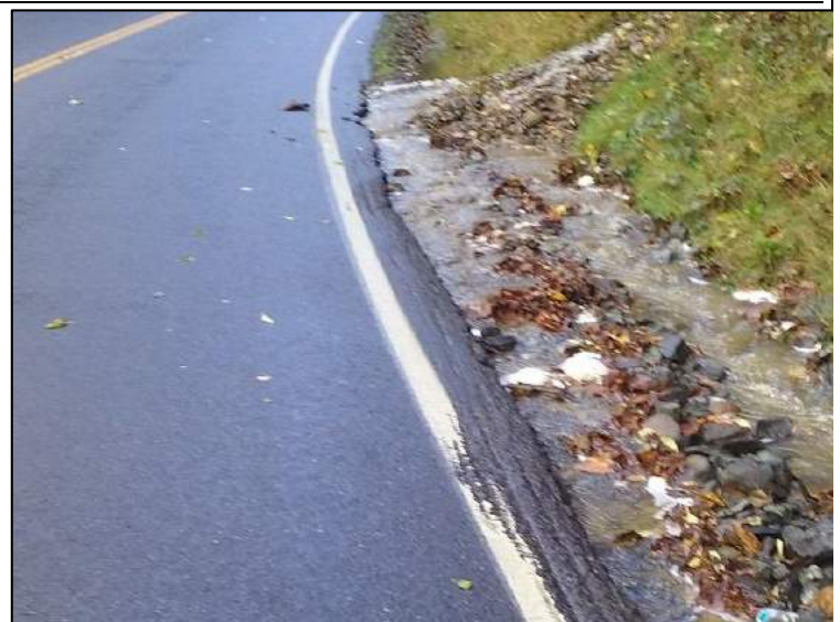
Stormwater along Jovita Boulevard
