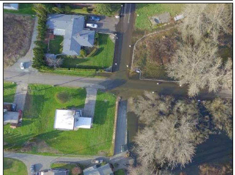
Flooding at Lake Chalet pothole
