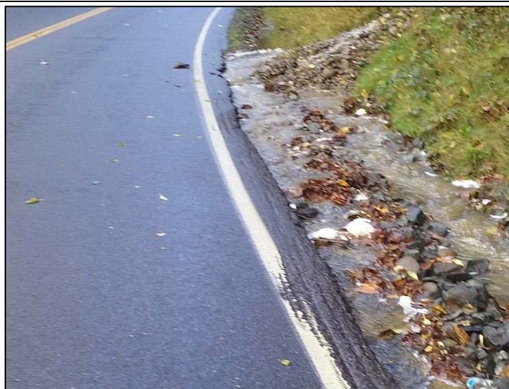
Stormwater along Jovita Boulevard
