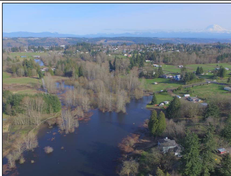
Edgewood Bowl pothole flooding
