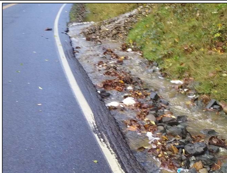
Stormwater along Jovita Boulevard
