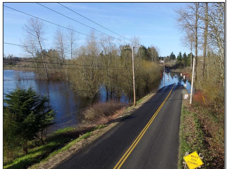
Edgewood Bowl pothole flooding
