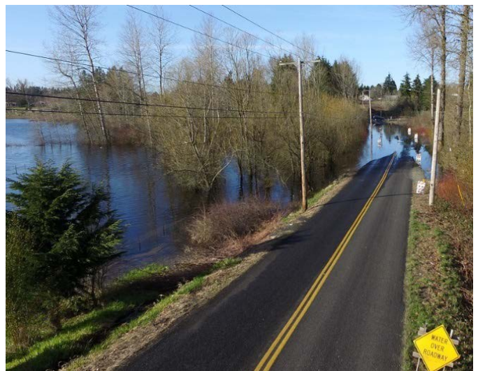
Flooding of the Edgewood Bowl Pothole causes road closures.
