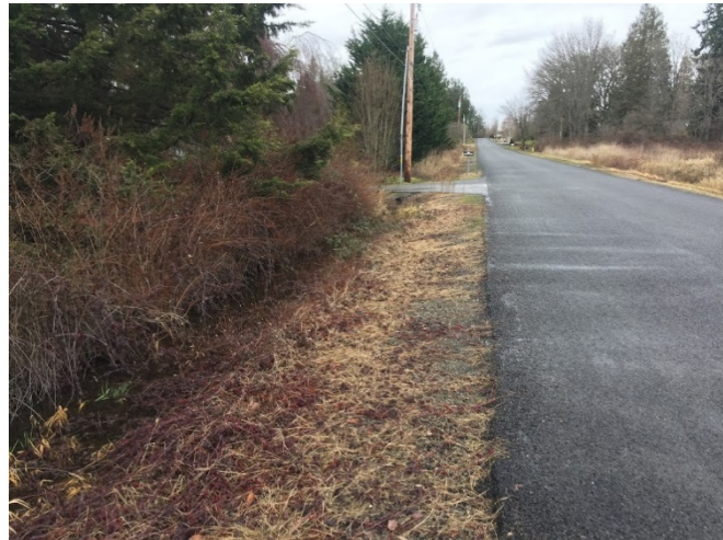
Roadside ditches that are part of the City's surface water conveyance infrastructure require regular maintenance.
