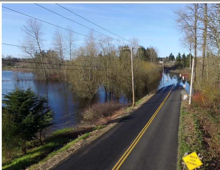
Edgewood Bowl Pothole flooding
