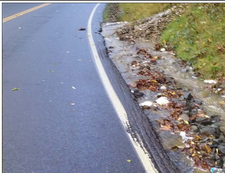
Stormwater along Jovita Boulevard
