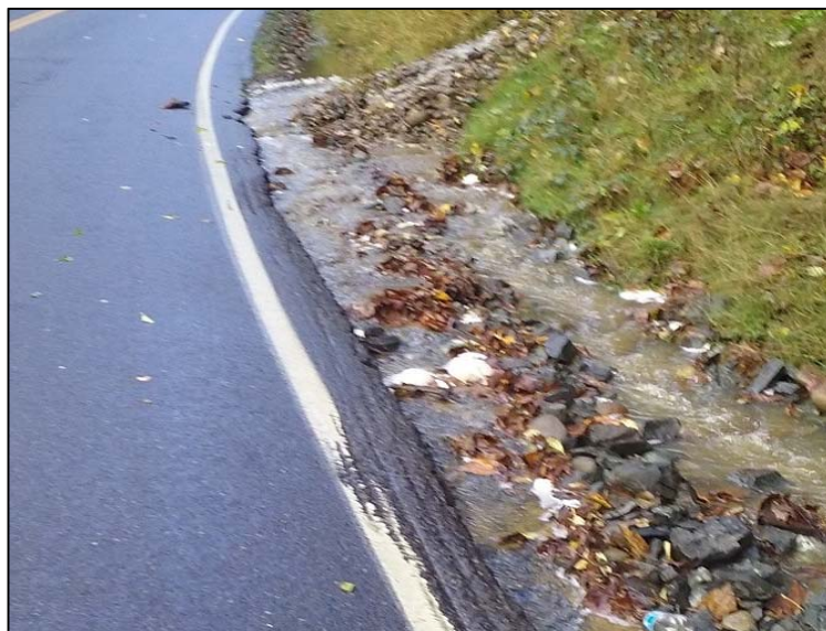
Stormwater along Jovita Boulevard
