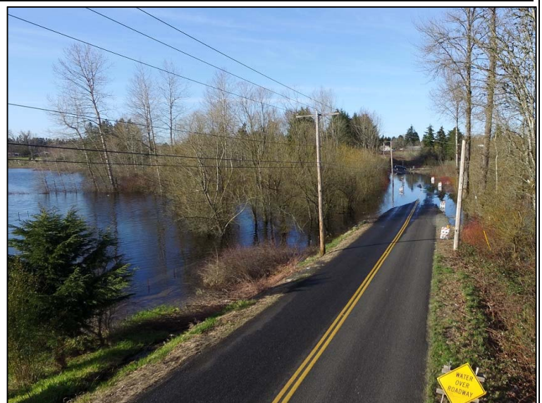
Edgewood Bowl pothole flooding
