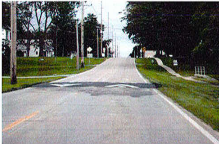
Figure 8. Driver view of speed table in Gilbert.
