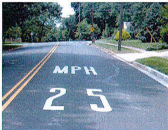
Special pavement marking to encourage speed reduction for impending curve.
