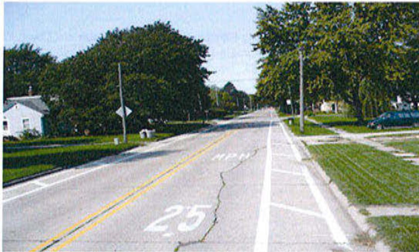
Figure 6. Shoulder markings used to narrow travel lanes in Roland.
