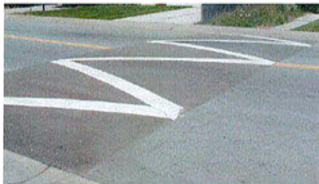
A speed hump delineated to notify motor vehicles of its presence.
