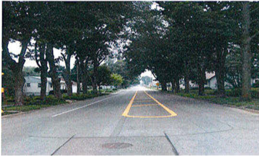
Figure 4. Painted center island and edgeline used to narrow lane.
