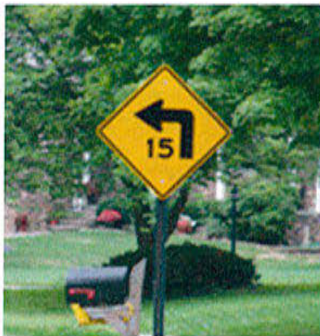
Advisory speed displayed with curve warning sign.
