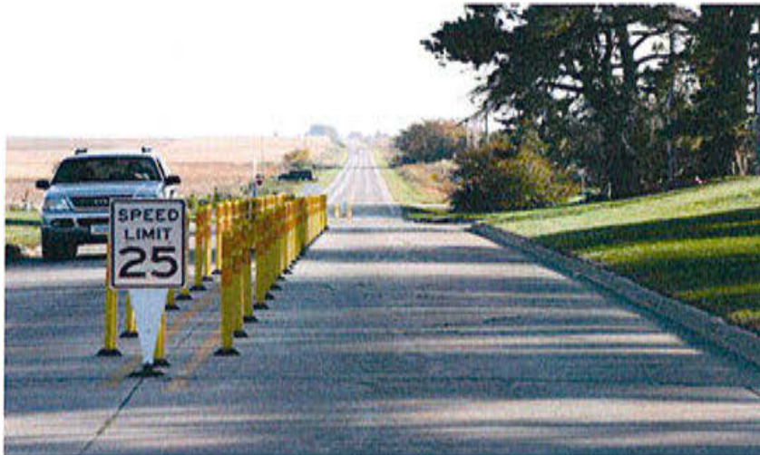
Figure 9. Tubular channelizing markers used for center island to narrow lanes.
