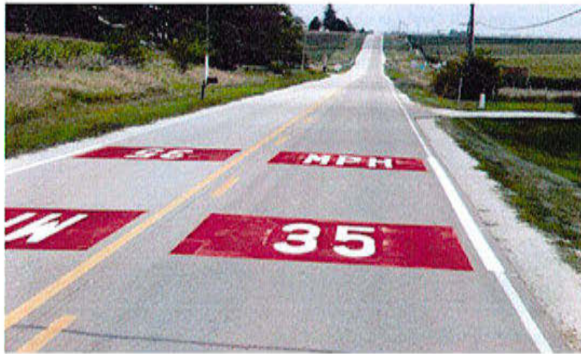
Figure 12. Speed limit markings with experimental red background in Dexter.
