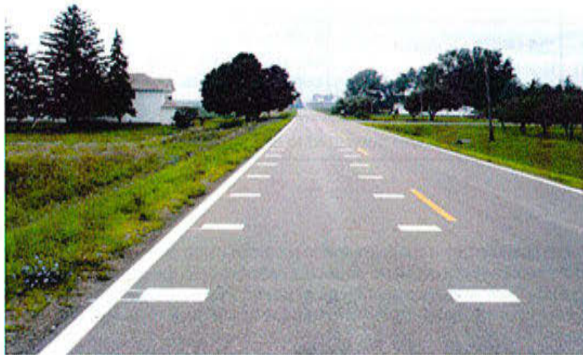
Figure 1. Experimental transverse markings at entrance to Union.
