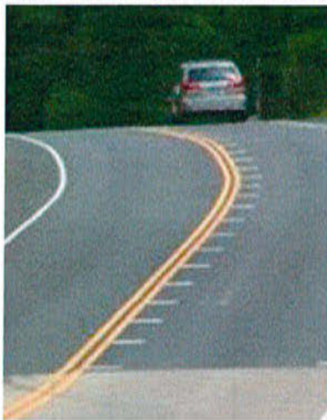
Optical speed bars on a rural roadway placed in advance of a horizontal curve.
