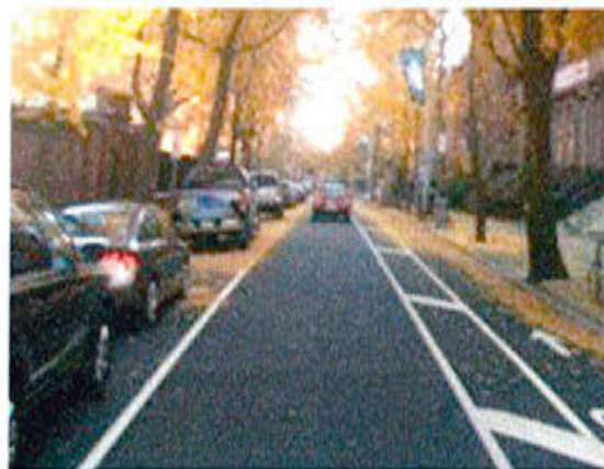
The lane width for motor vehicle travel in this community was reduced to provide exclusive space for cyclists.
