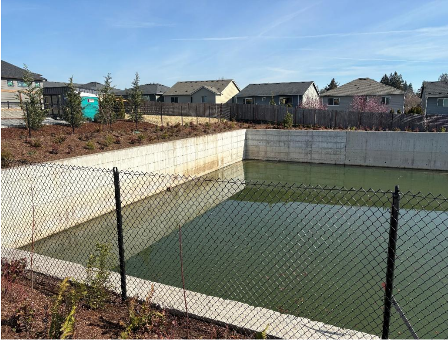
Stormwater Retaining Wall Example:
