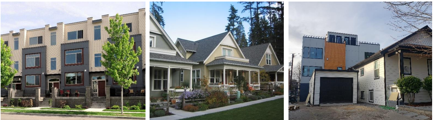
Left to right: Townhouses in Spokane, cottage housing in Kirkland, and a fourplex built behind an existing single-family residence in Seattle
