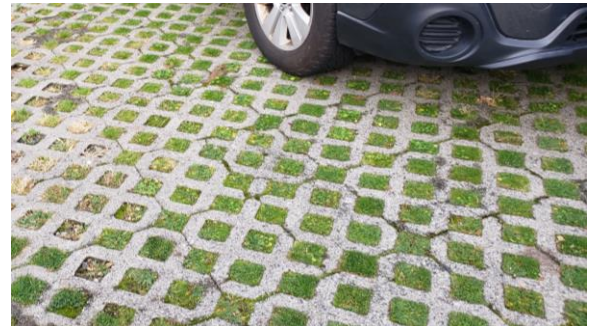
Figure 3. Example of grass block pavers at a residential development. Photo by MAKERS.
