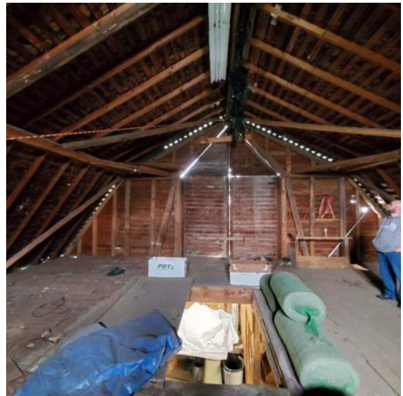
Photo: 3.2.5.4: A view of the loft space
