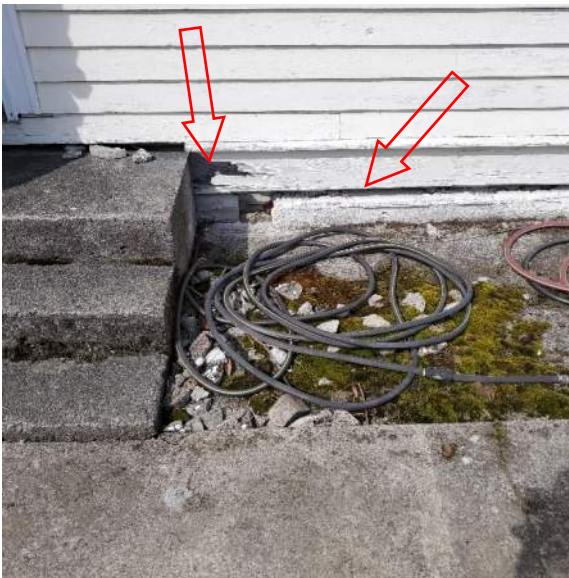
3.4.5.3 The floor structure has rotted out and there is an air gap between above the foundation wall.
