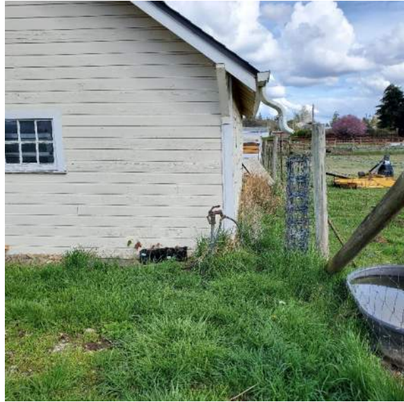
3.5.6.2 The structure is out of plumb. It is more noticeable at the windows and window frame.
