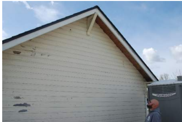
3.5.6.4 Paint blistering and peeling on the east facade
