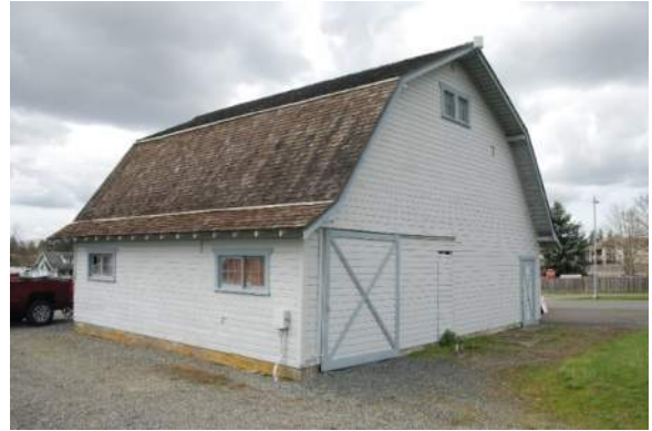
Photo 3.2.5.2: The rear façade of the barn
