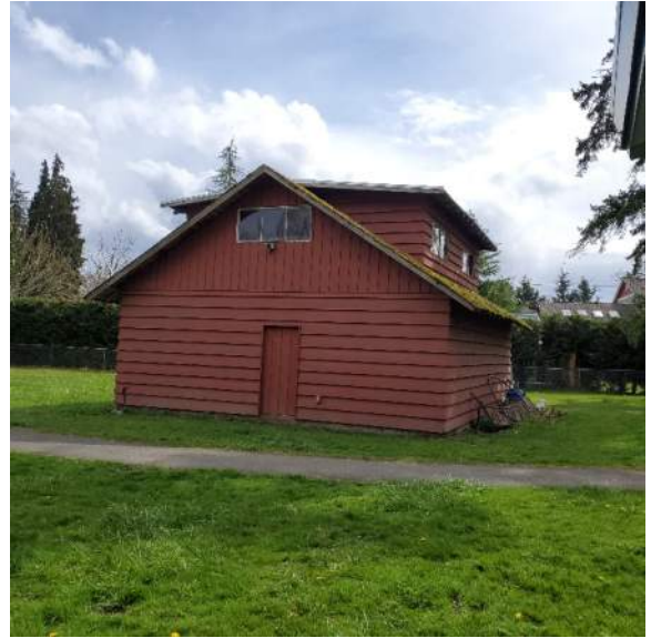
3.3.5.2 The north elevation with a man-door.
