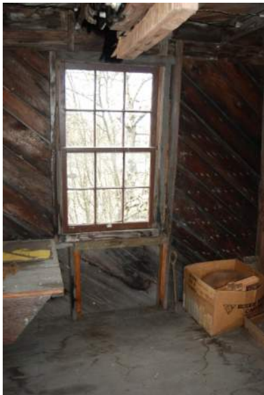
Photo 3.1.5.3: An interior view of the window.
