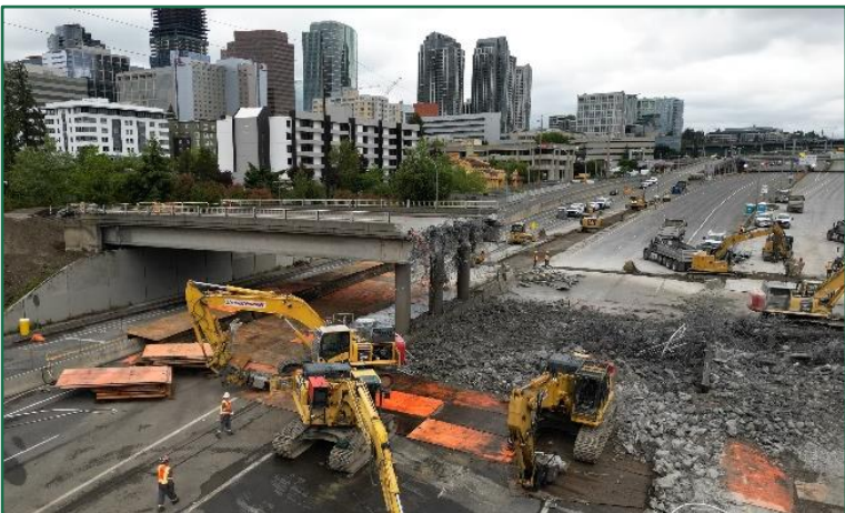
Main Street Bridge Replacement
