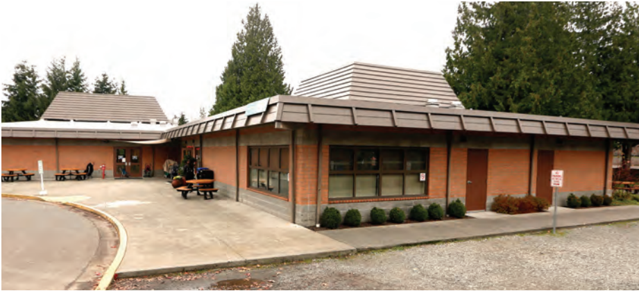
Shoreline Community College: Left: New sheet metal mansard roof; Right: Existing cement shingles
