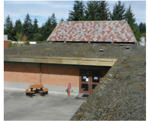
Shoreline Community College: Left: New sheet metal mansard roof; Right: Existing cement shingles
