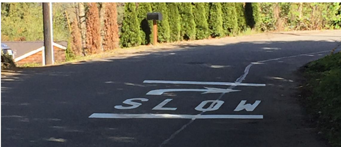
Figure 1 – SLOW with arrow on-pavement marked legend
