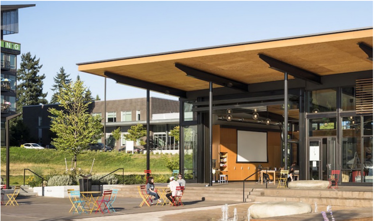
The Hangar at Kenmore Town Square uses natural colors and a variety of wood, glass, metal, and other materials on the interior and exterior.
