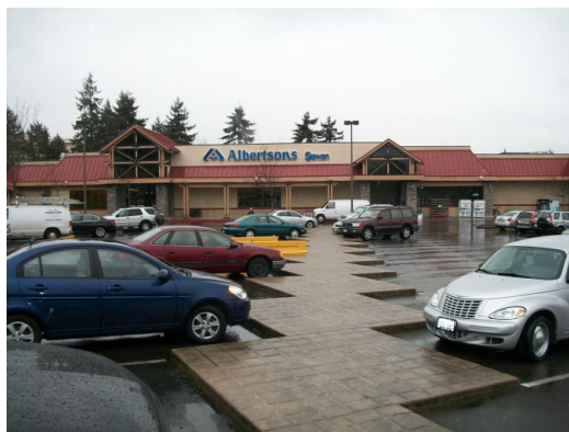
Figure 24 – Pedestrian path through grocery store lot that is separated from vehicle use areas.
