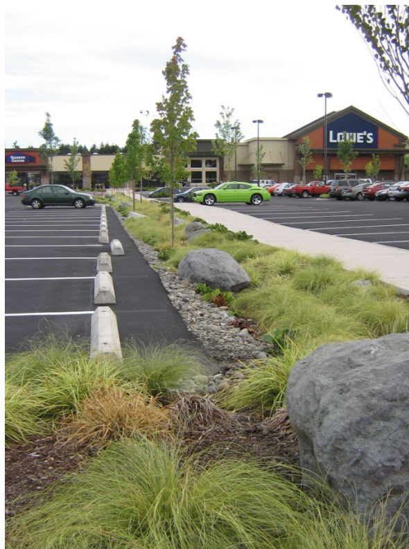
Figure 29 – Low impact development stormwater facility integrated into parking lot design and pedestrian circulation concept of a large format retail site is highly functional and enhances the overall aesthetic appeal.
