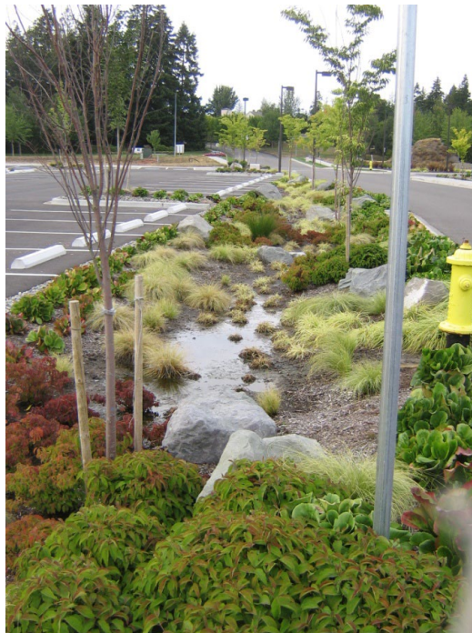
Figure 12 – Parking lot featuring smaller parking areas, significant landscaping and integrated low impact development stormwater facilities.
