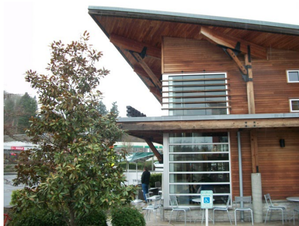
Figure 51 – Weather protection built into building design.
