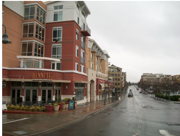
Figure 42 – Apparent building mass is reduced through varied roof forms, step-backs and individual storefronts.
