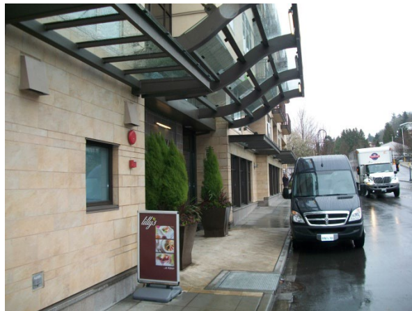
Figure 52 – Weather protection attached to building.
