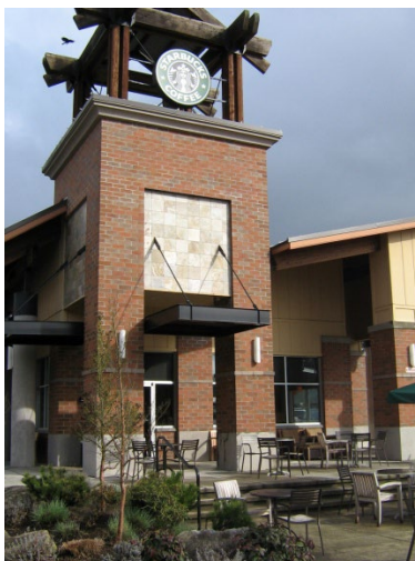
Figure 18 – Corner treatment with public space, architectural feature and landscaping creates an inviting entry and place for social activity.
