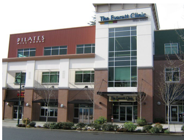
Figure 39 – Facade showing changes in materials, distinct window patterns, changes in color, and articulation.
