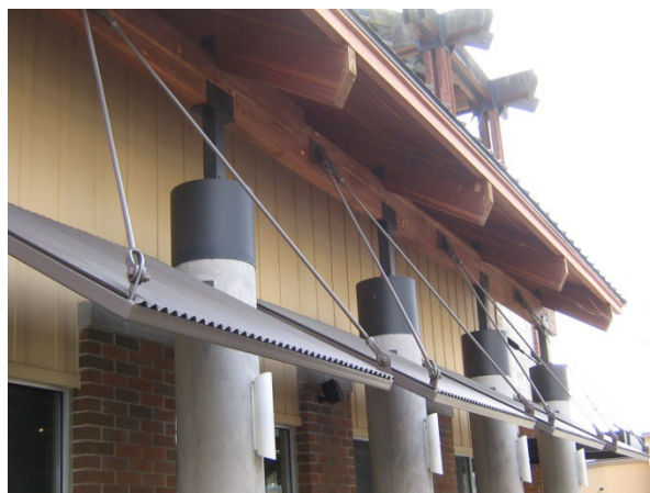
Figure 53 – Building material detail showing durable materials and changes in materials creating variation.
