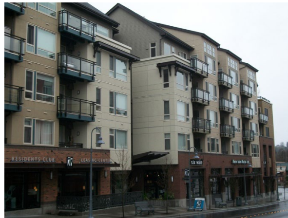
Figure 40 – Building articulation, changes in materials and separated roof forms.
