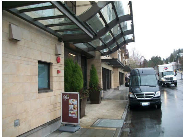
Figure 52 – Weather protection attached to building.
