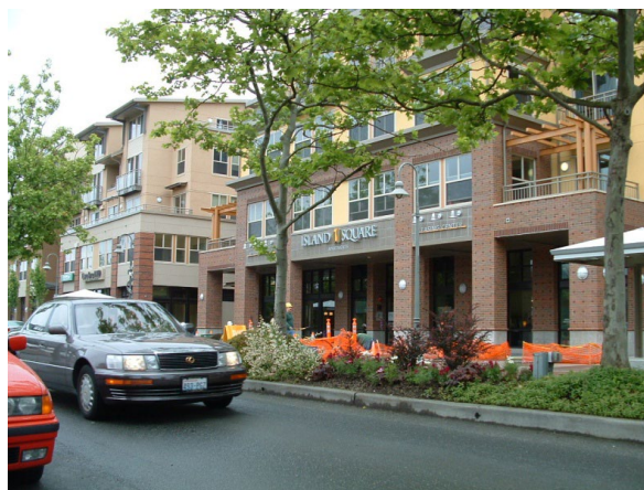
Figure 38 – Building articulation and changes in materials reduce the apparent bulk of the structure.
