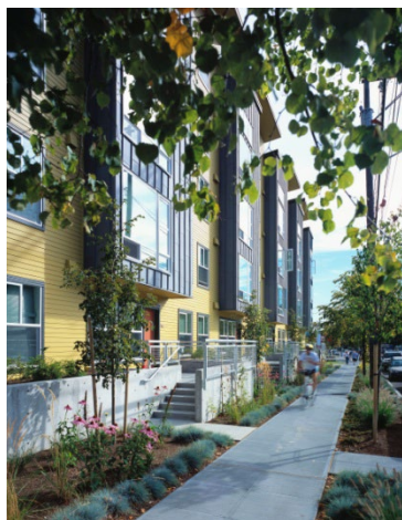
Figure 8 – Residential sidewalk showing clear walkway area and substantial landscaping for visual interest.
