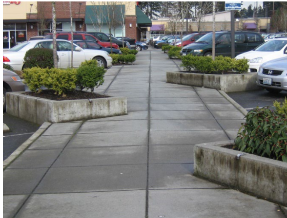
Figure 22 – Pedestrian access route through parking area separated by curb and distinctive pavement.
