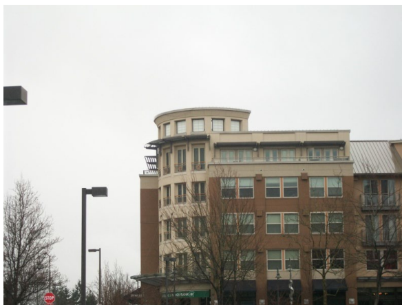
Figure 56 – Raised parapet wall to screen roof mounted mechanical equipment.
