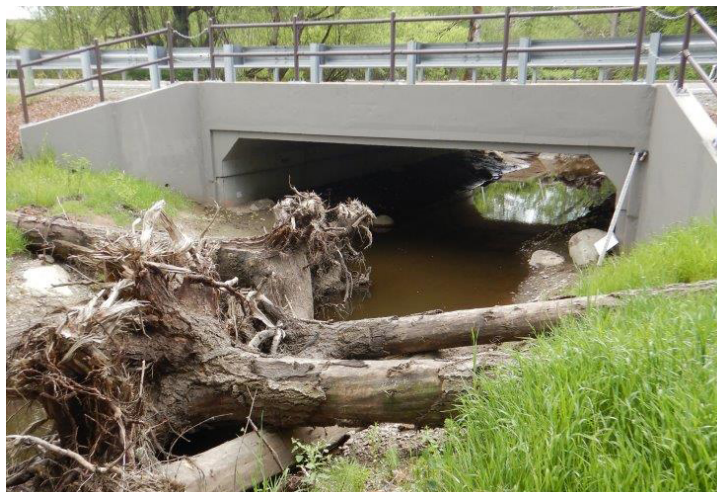
After: New structures at tributaries to Patterson Creek allow all fish of all life stages to pass through unimpeded. Large woody material gives fish access and habitat to swim, eat, rest, and spawn as needed.
