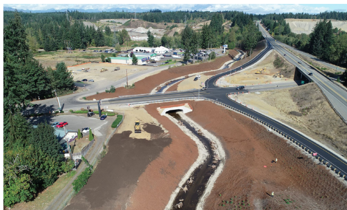
After at Coffee Creek: the newly aligned channel opens up over 13 miles of habitat and eliminated a county barrier downstream making the structure immediately accessible to fish.
